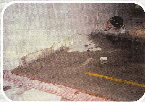
COLD JOINT REPAIR — BEFORE
