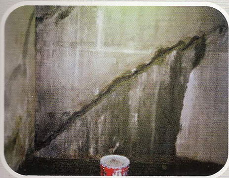
CRACK REPAIR DAY ONE
