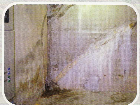
CRACK REPAIR DAY SEVEN
