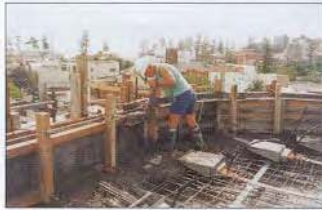
FIGURE 10 - CAST IN-SITU PARAPETS
