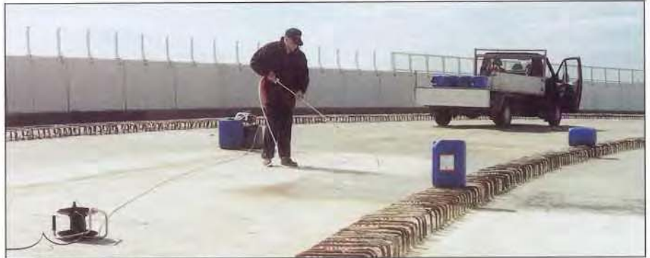
RADCON #7 - APPLIED TO STRUCTURAL CONCRETE
