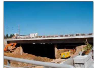
FIGURE 14. Works on Gaia Bridge
