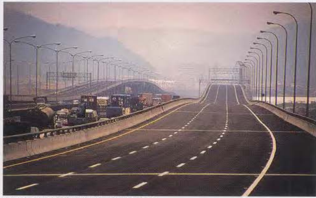
PHOTO 8 - FINISHED FREEWAY COVERED IN ASPHALT TOPPING
