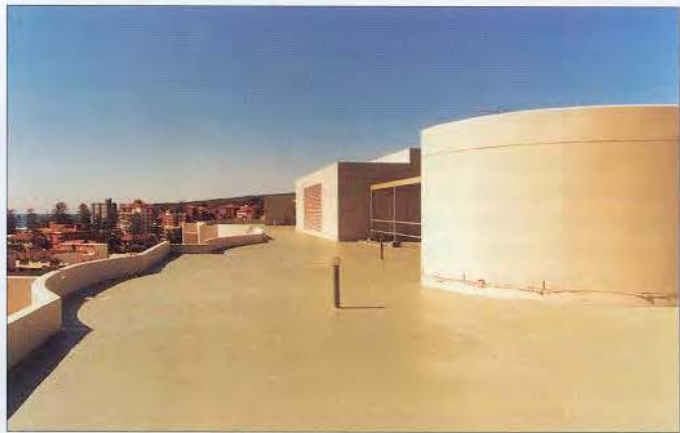
FIGURE 13 - RADCON #7 TREATED FIRST, THEN PAINTED
