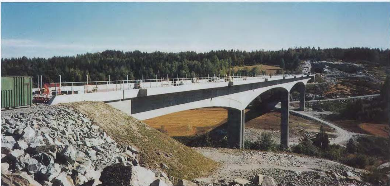
FIGURE 14 - HOLENDALEN RAILWAY BRIDGE, NORWAY
