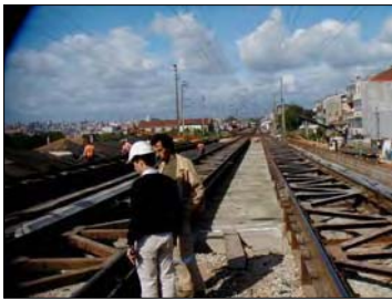
FIGURE 11. Inspecting the structure before waterproofing
