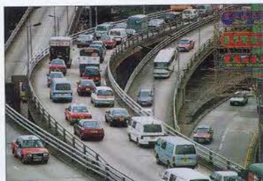
FIGURE 11 - CLOSE UP OF OVERPASS
