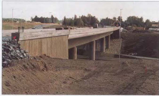
FIGURE 29 - KVERNDALEN BRIDGE, NOOSDLO
