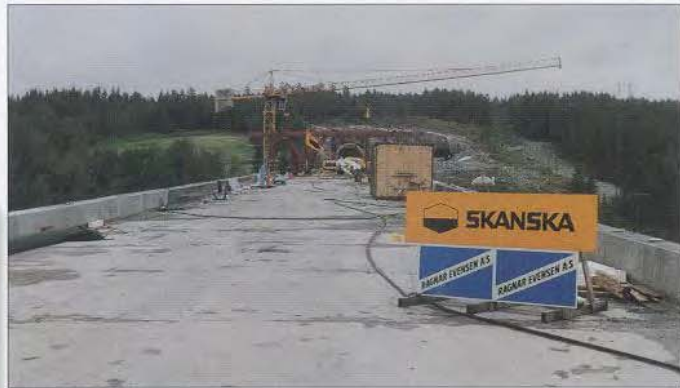
FIGURE 15 - BRIDGE DURING CONSTRUCTION
