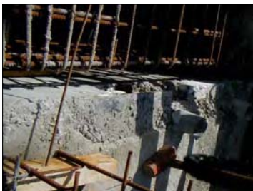
FIGURE 12. The reinforcement works
