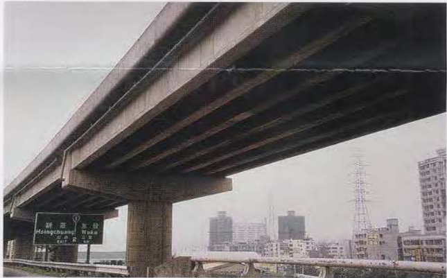
PHOTO 9 - UNDERSIDE OF RAISED FREEWAY
