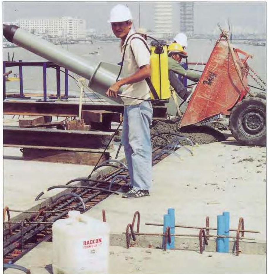
RAMA VIII - PRE-CAST PANEL JOINTS
