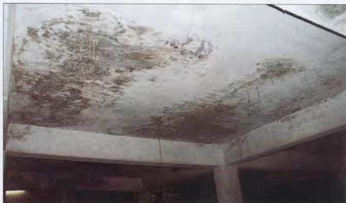
FIGURE 31 - SOFFIT WITH 300MM CALCIUM STALACTITES
