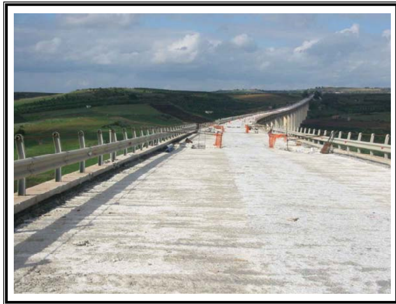
Raised Highway SS115 - Italy
