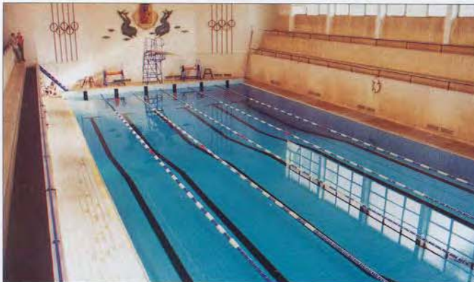
FIGURE 30 - SWIMMING POOL RE-FILLED AFTER SUCCESSFUL REPAIRS
