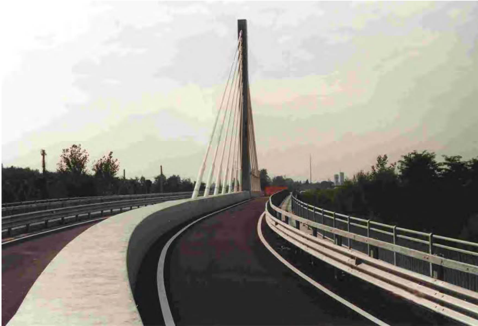
Bridge over Livenza river, (TREVISO) - 1.600 Sqm Waterproofing with RADCON #7 of the bridge deck.
