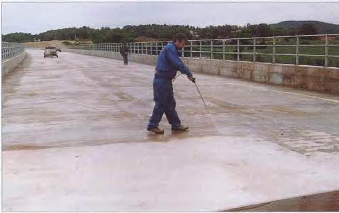
FIGURE 24 - RADCON #7 APPLICATION
