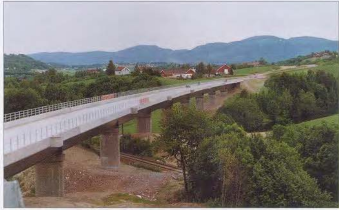
FIGURE 25 - BREMSA BRIDGE, NORWAY
