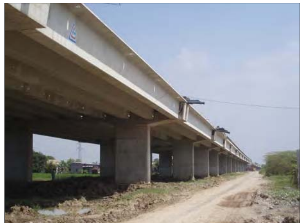
FIGURE 2. Part of the Super Highway currently under construction
