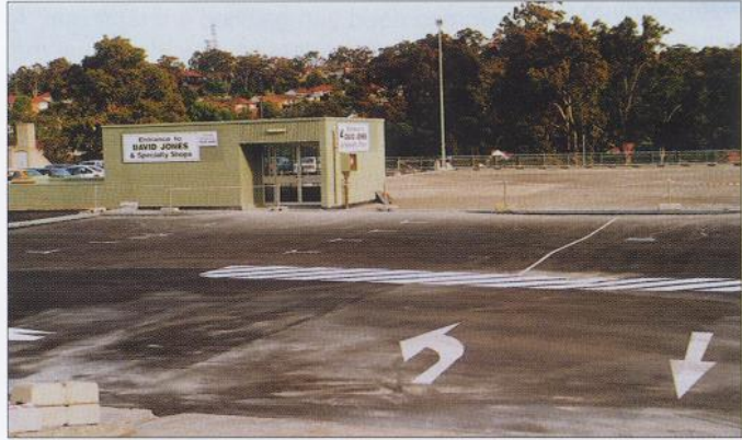
TOP DECK OF CAR PARK
