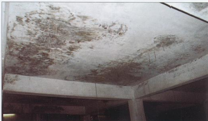
FIGURE 31 - SOFFIT WITH 300MM CALCIUM STALACTITES
