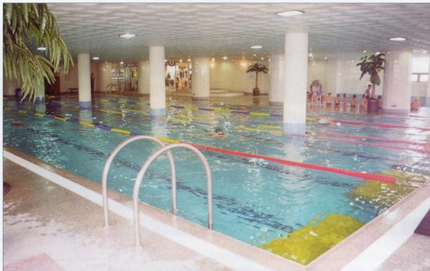
FIGURE 43 - MAIN SWIMMING POOL WATERPROOFED WITH RADCON #7
