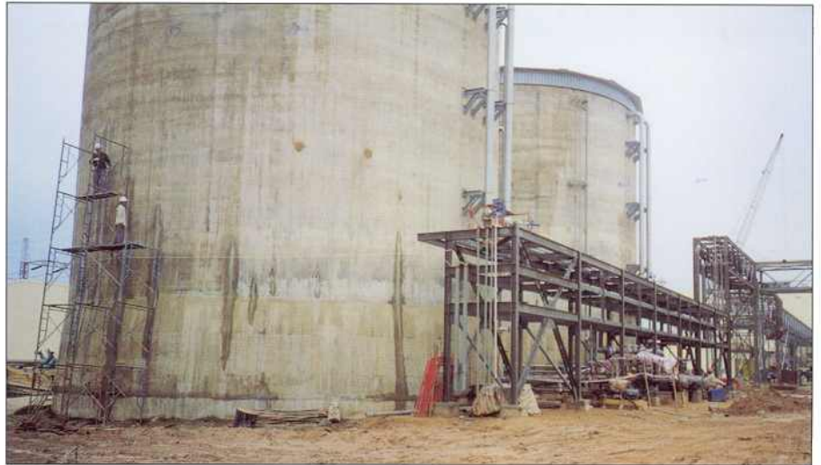
WATER TANKS - POWER PLANT - 6000 SQ METRES
