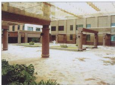
FIGURE 5 - PODIUM LEVEL COMPLETED
