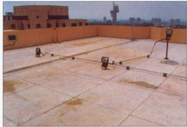
FIGURE 24 - ROOFTOP WITH INSULATION AND TOPPING
