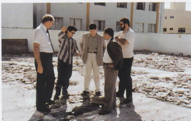
PHOTO 13 - TILES BEING REMOVED TO REPLACE FAILING MEMBRANE
