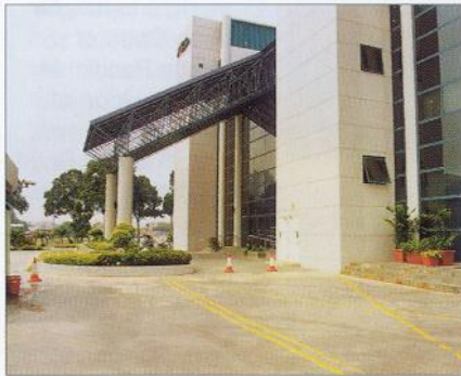
FIGURE 41 - ENTRANCE SUSPENDED OVER BASEMENT
