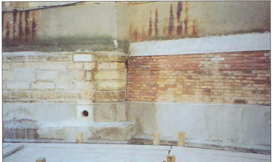
VENICE CANAL RESTORATION
