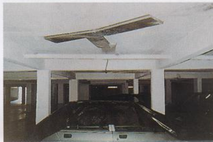
PHOTO 14 - GUTTERS USED AS SHORT TERM SOLUTION
