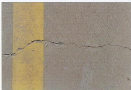
FIGURE 30 - ONE OF MANY CRACKS IN THE DECK
