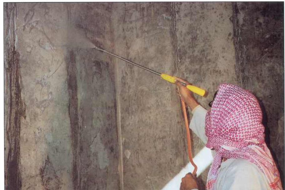
WATER TANK – ABU DHABI
