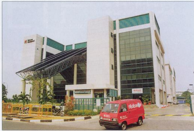
FIGURE 42 - TELECOM EQUIPMENT BUILDING, SINGAPORE
