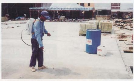
the construction timetable. Once Radcon #7 is applied, the area becomes trafficable within a matter of hours, after the first watering procedure is concluded.
