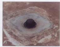
the fulgo inlet received a RX Waterstop from American Colloid as detailed in Figure 22 & finished in Figure 23.
