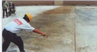
centre. With the correct site preparation and large unobstructed areas of rooftop, application rates up to 4,000 square metres per day were achieved with one motorised spray unit.
