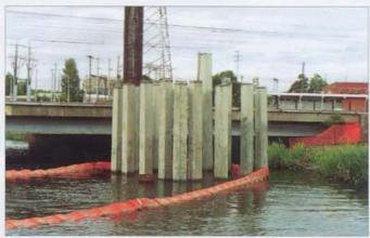
FIGURE 39 - PILES DRIVEN INTO MOONES PONDS CREEK
