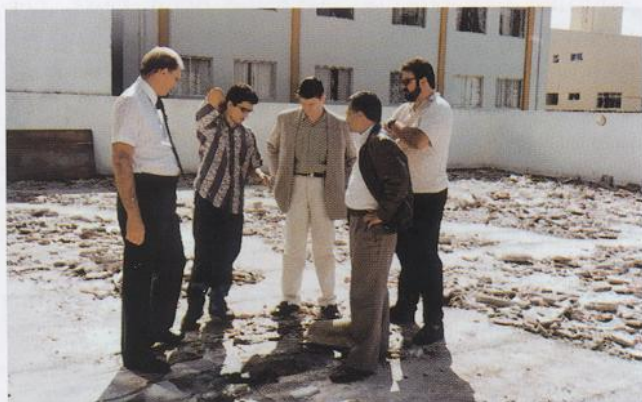
PHOTO 13 - TILES BEING REMOVED TO REPLACE FAILING MEMBRANE
