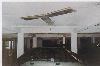
PHOTO 14 - GUTTERS USED AS SHORT TERM SOLUTION
