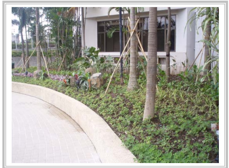
Figure 2: Radcon Formula # 7 is now waterproofing and protecting these planter boxes
