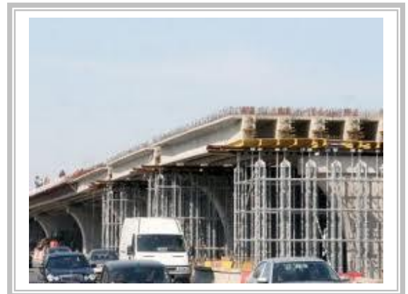
Figure 2: Construction of Baneasa Underpass
