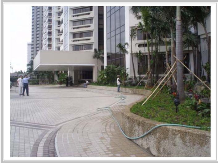
Figure 1: Entrance to Ritz Towers
