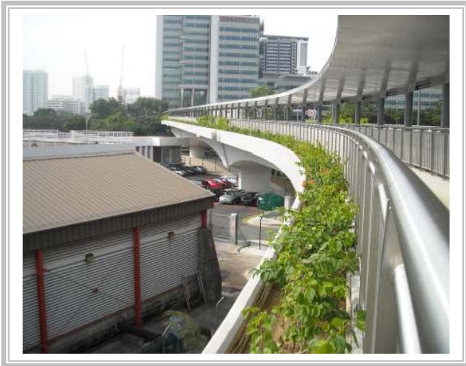
Figure 1: Planter boxes on the bridge
