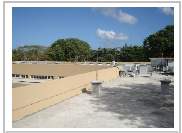
Figure 2: Roof of Technical Building
