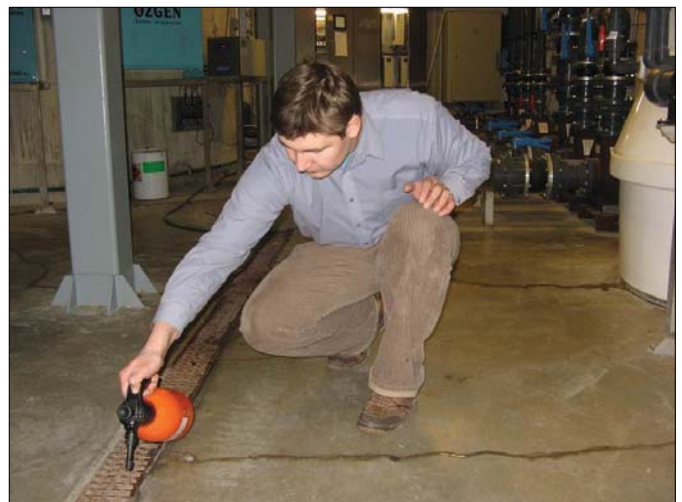
FIGURE 2. Porto Stavba applicator Mr Edgaras Kaveckas sealing all visible cracks with RADCON #7 prior to the treatment.
