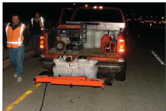
Pictured above: RADCON Formula #7 application - electrical pump/tank with a hose spray wand or a boom with a number of sprayers.
