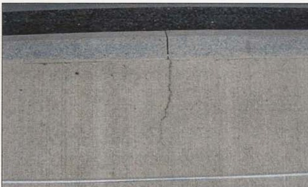
FIGURE 5 & 6 Cracks on the drainage areas
